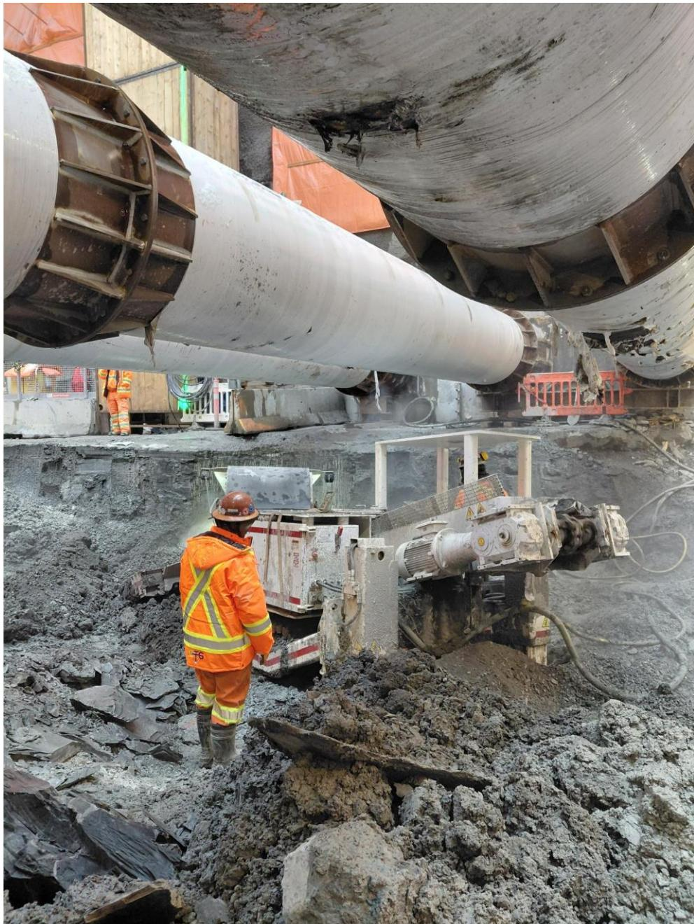
*The final stages of excavation are underway at the Queen-Spadina south site, using a roadheader to minimize impact to the community.*
