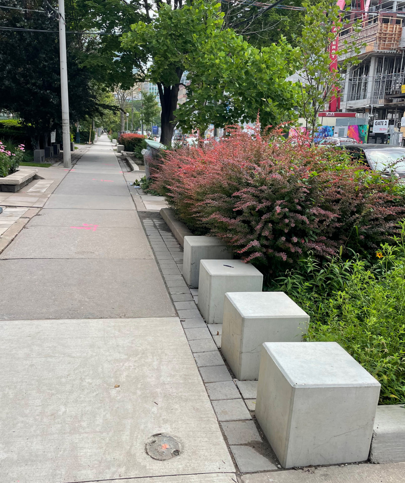
Existing conditions on Wellington Street West
