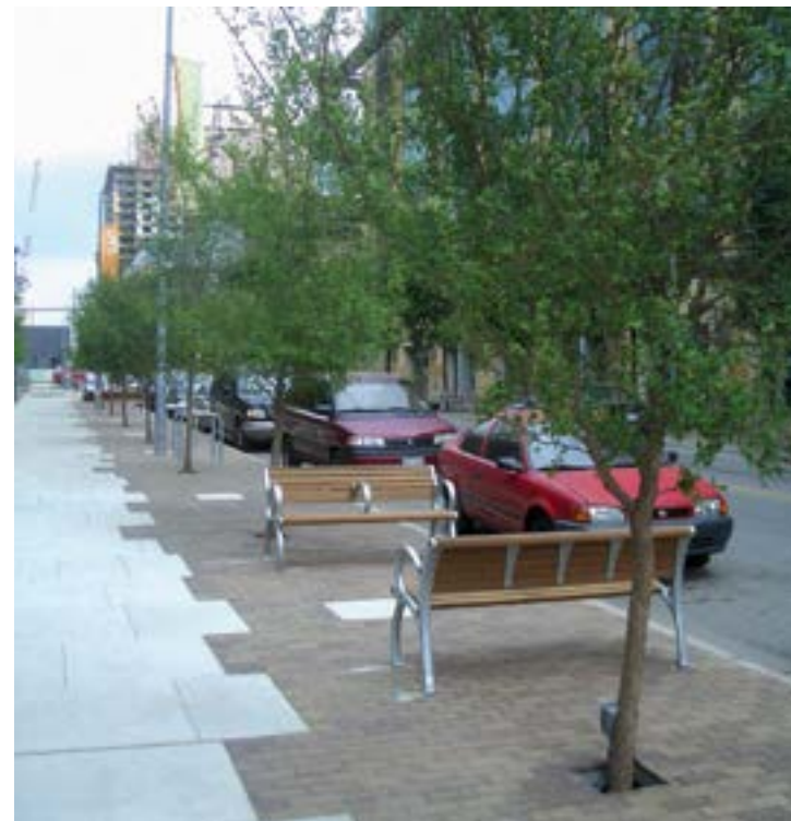
Example of a widened sidewalk on one side of the street in Austin
