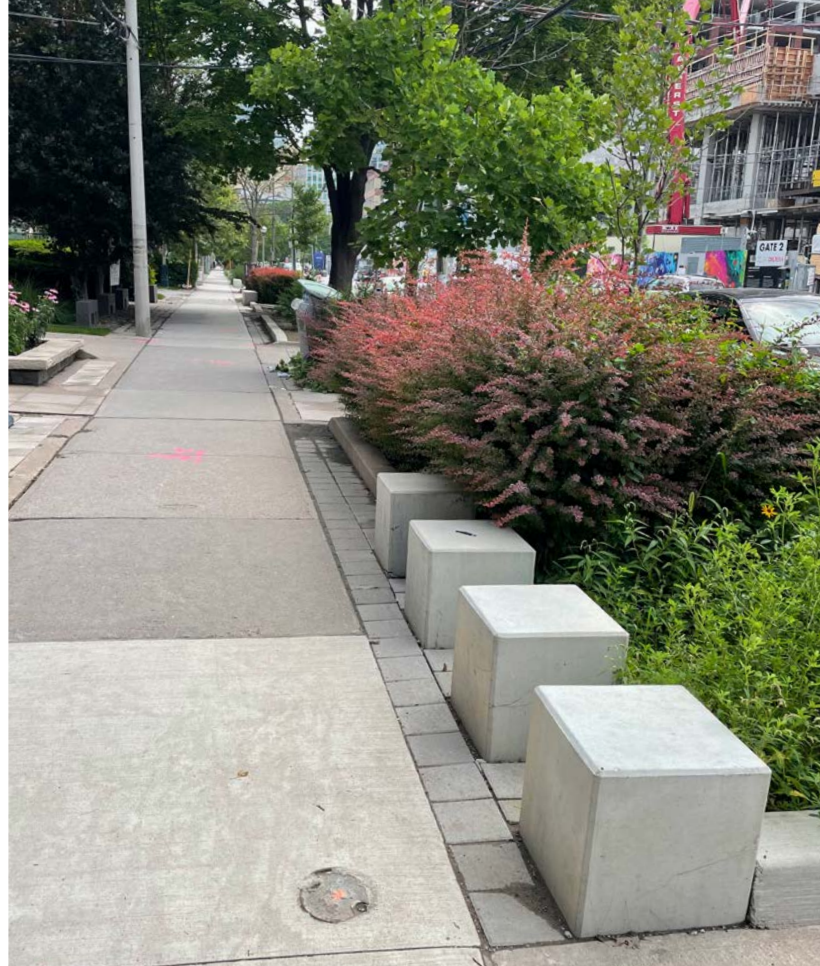
Existing conditions on Wellington Street West
